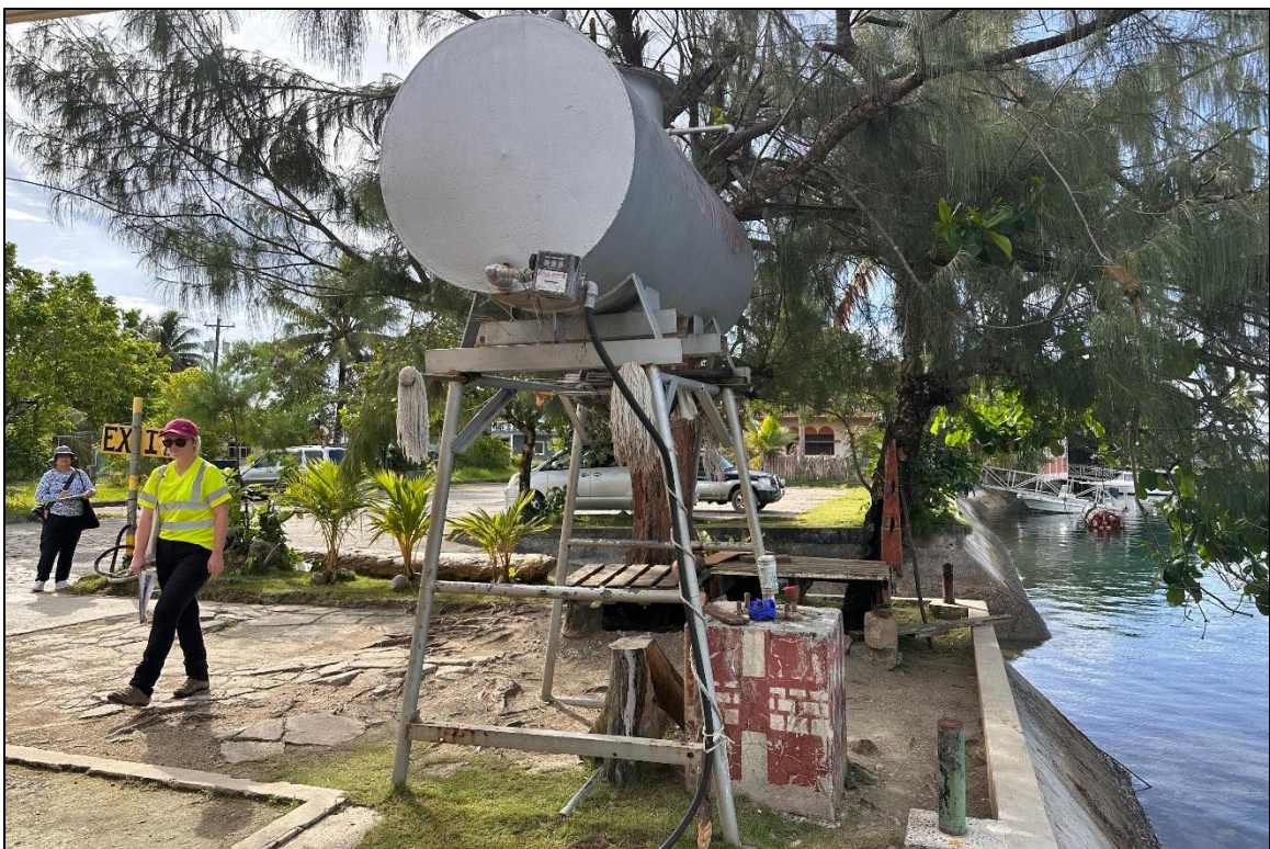
Photo 28: Overview of 320-gallon kerosene AST lacking secondary containment. Photo is looking east.
