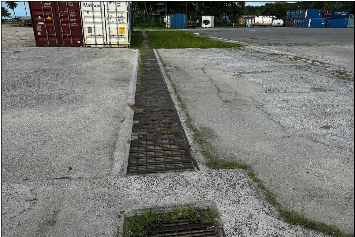
Photo 11: Storm drain channel which encircles the gated area within the port and leads toward the ocean. Photo is looking south.
