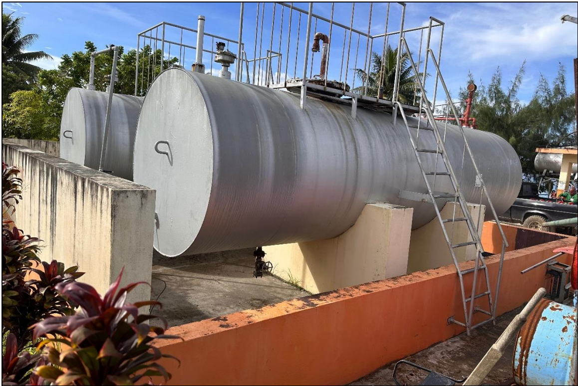
Photo 27: Overview of two steel ASTs containing diesel (3,700 gallons) and unleaded gasoline (4,010 gallons) in a concrete secondary containment observed at YCA Rufan Gas Station. Photo is looking north.
