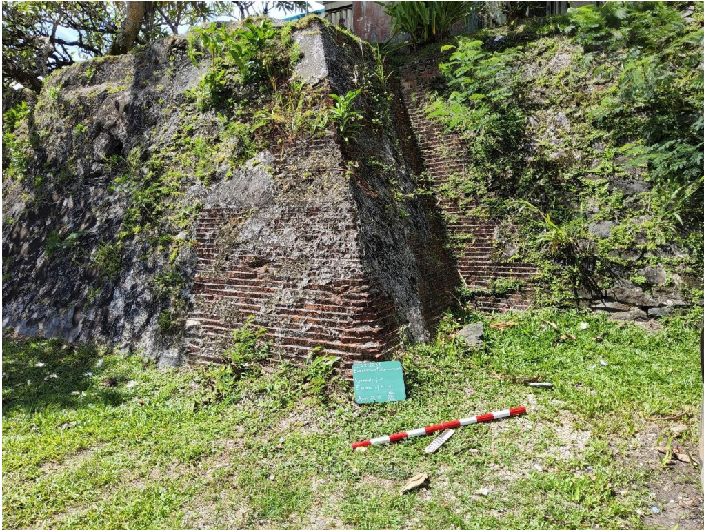
Figure 3-17 Feature 06, Northeast Corner Built of Coursed, Mortared Brick; View Facing Southeast; Note the Remnant Plaster
