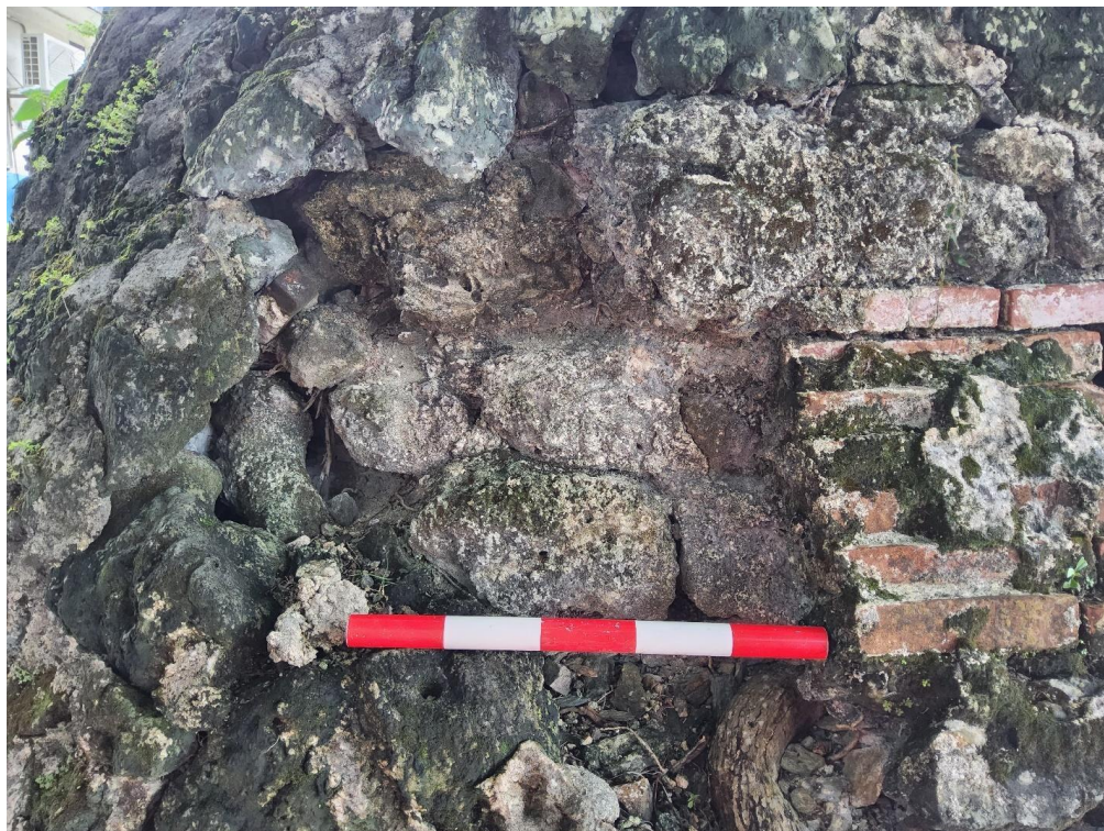
Figure 3-16 Feature 06, Detail of the Southeast Corner Showing Rubble (Left), Rough Ashlar (Center), and Brick (Right) Construction; View North
