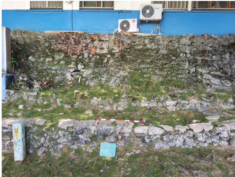
Figure 3-22 Feature 06, Section of the South Wall Damaged and Rebuilt Using Original Spanish Brickwork Fragments; View North
