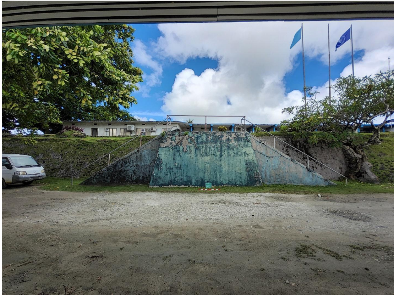
Figure 3-4 Feature 01 Overview, a Pair of Large Concrete Staircases Built along the East Side of the Spanish Fort during the Japanese Administration; View West; Staircases Built against Feature 06, the Spanish Colonial Earthen and Masonry Embankment
