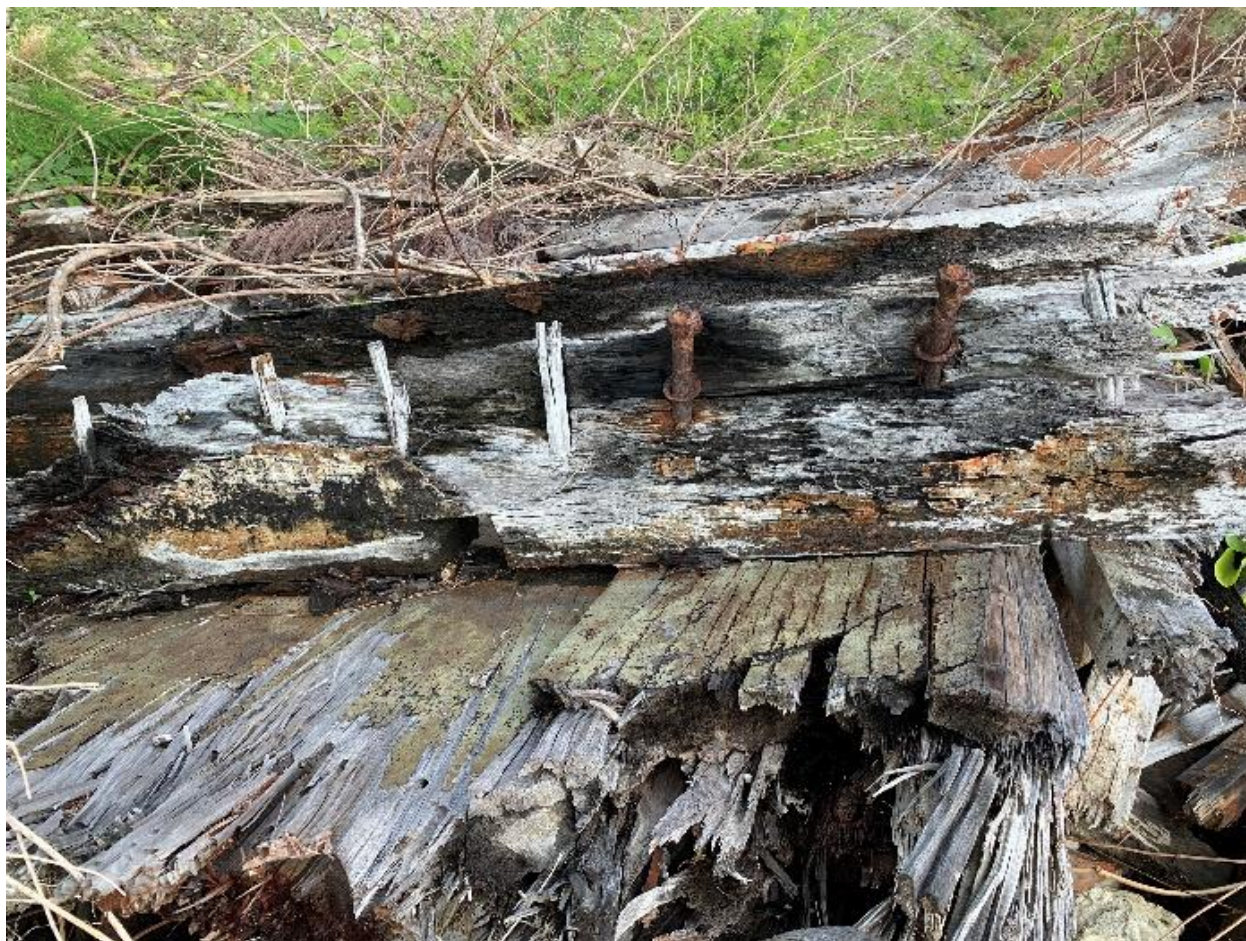
Figure 3-78 Treenails and Iron Bolts (Photo by AECOM)
