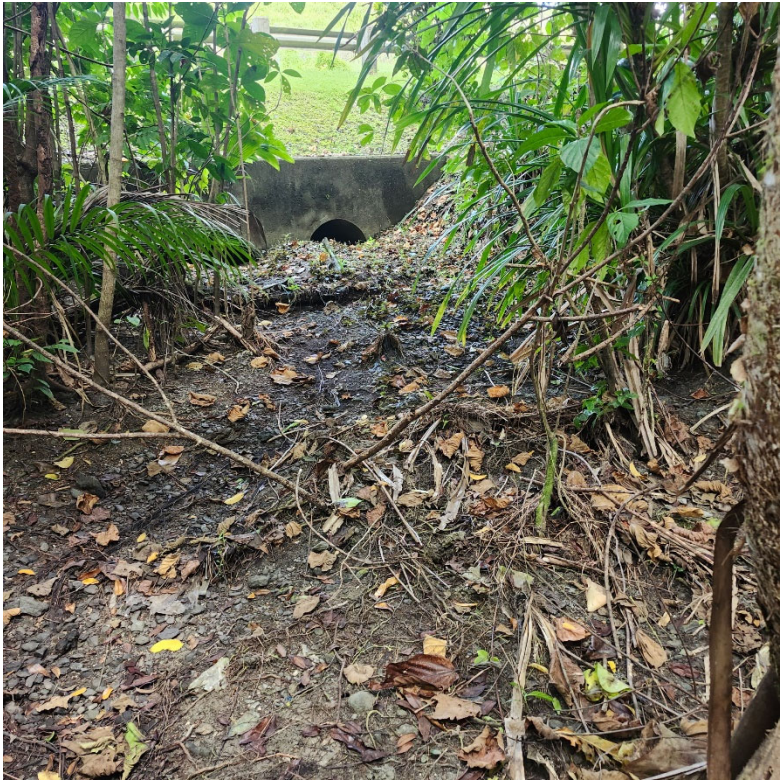
Area 5, Culvert with a drain flowing toward Wetland 18.
