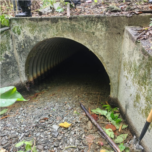
Area 5, Culvert near wetland 22.
