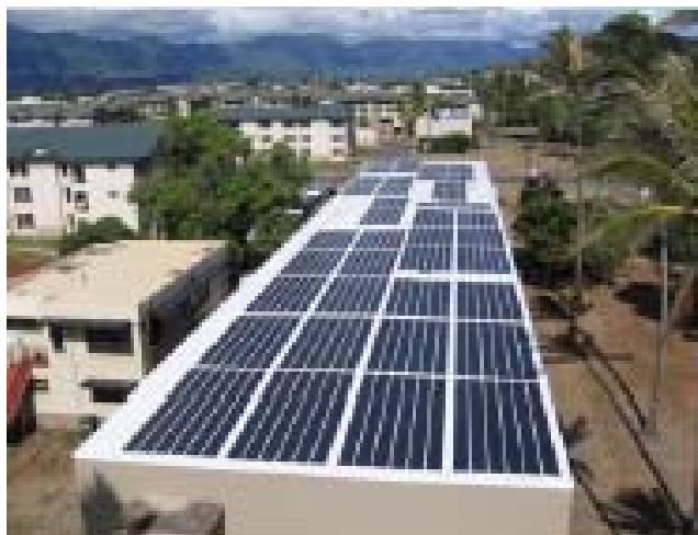
An example of a renewable energy project is this Building Integrated Photovoltaic (BIPV) rooftop on a barracks at Kaneohe Marine Corps Base, Hawaii
